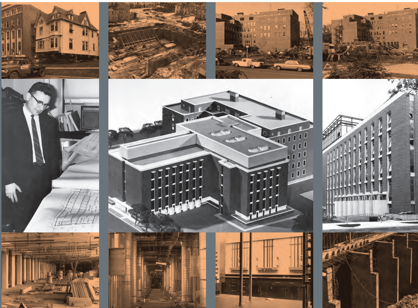
Roger Adams Laboratory: various stages of planning and building.
